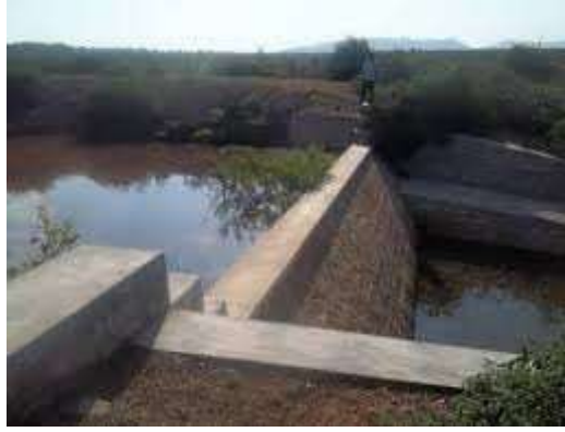
Figure 6. A check dam in Rajasthan.
